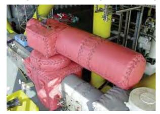
Darmatt TM - a unique flexible, passive fire protection system that can meet 180 minutes blast protection up to 0.43 bar, protecting personnel and providing asset protection. DARMATT provides protection for valves, actuators, cable routes, conduits signal lines, junction boxes, solenoid stations, air receivers, process vessels and other equipment applications requiring fire protection.
